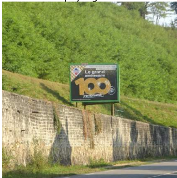
Avenue Baudin Valin
